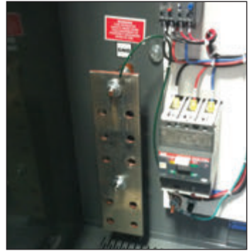
Figure 3 Main Load Bus
