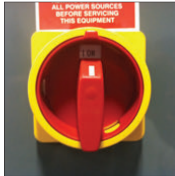
Figure 20 Fan/Control Power Disconnect Switch
