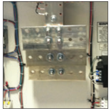
Figure 3 Main Load Bus
