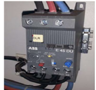
Overload Relay (OLR)
