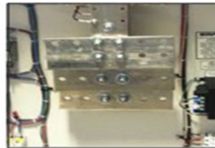
Bottom view of a Mars, showing removable plate for cable connections.
