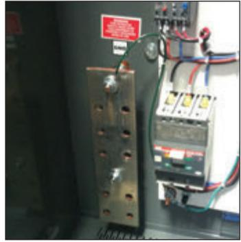
**Figure 4 Main Load Bus**
